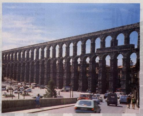
The aqueduct, built without mortar, has 166 arches
